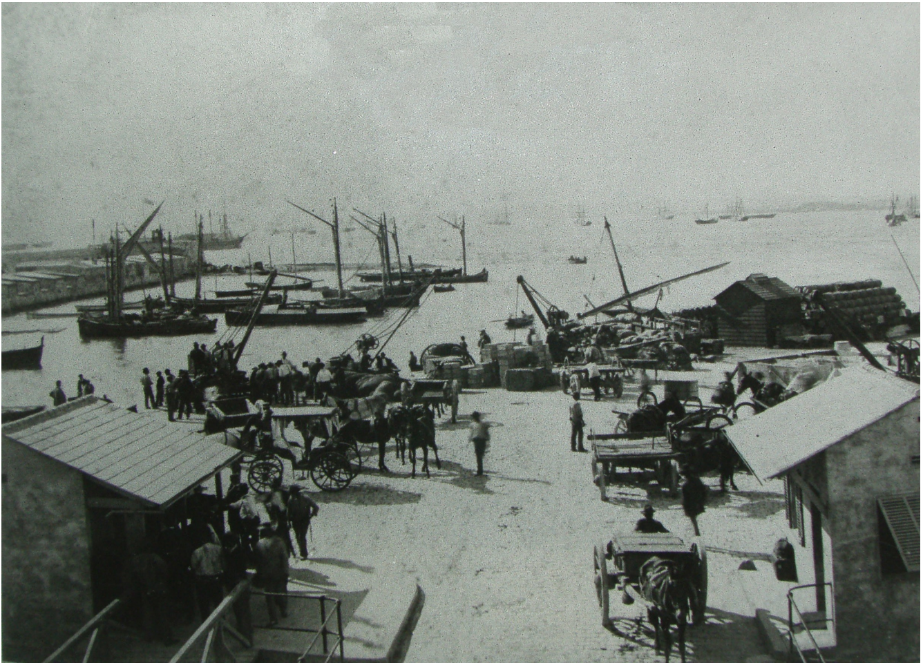
Landport Wharf, 1878, showing in the foreground the customs and police controls and, in the distance, coal hulks
